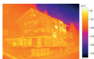
Image thermique sans testo ScaleAssist
